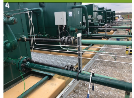
Modular EQUIPMENTGUARD base pads are easily moved into place and ready for immediate use.
